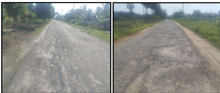
Improvements of Thunukkai - Thenniyankulam Road (0.000-1.000km)
